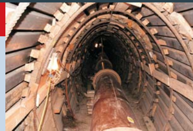
Figure 3: New installation of vitrified clay tubes
