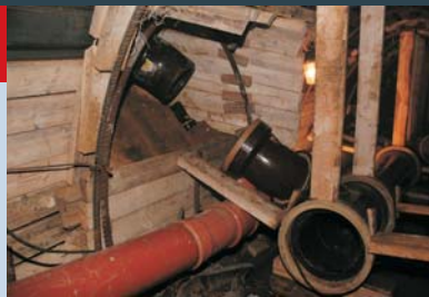
Figure 2: Horizontal galleries for side connections
